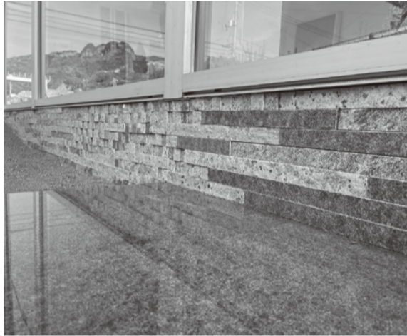
外壁は「Build with 庵治石」で施工
